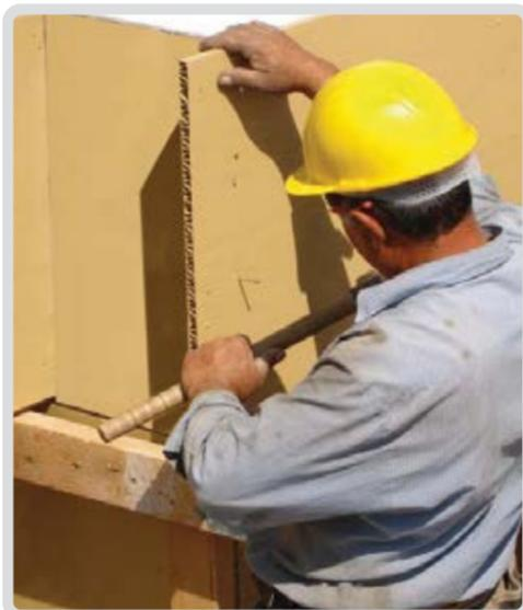
**5 -** Durable against nailing, drilling and cutting. For ideal application, it is recommended to use special wide capped Pladeck nail.
